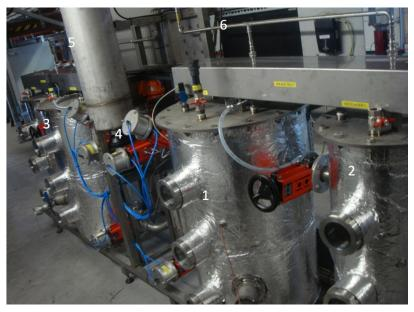
Figure 2: Partial view of the pilot plant installed at the DBFZ (Deutsches Biomasseforschungszentrum gGmbH) 1: digester 2, DD; 2: secondary digester 2; 3: digester 1, DB; 4: pneumatically operated slides V5 / V6; 5: homogenization tank; 6: biogas pipeline (© U. Pliquett)
