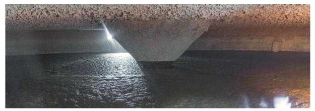
Figure 1: Inside view of the fermenter. Through microbial degradation of the hydrogen sulphide, deposits of elementary sulfur are deposited on the ceiling. © State Institute of Agricultural Engineering and Bioenergy, University of Hohenheim.
