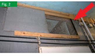
Manual additional air slide – view from central corridor, face upwards
