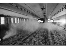
Fig. 1: Fans built in the gable wall
